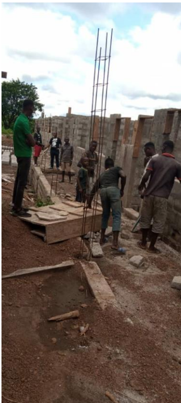
Bouw van school in Karene District.
